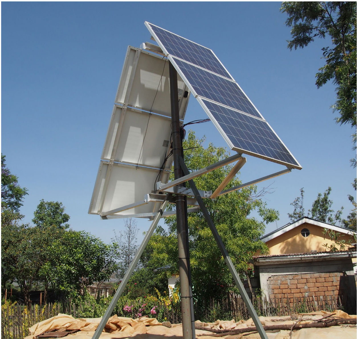
Powering Agriculture innovator SunDanzer’s East-West facing panels create a flatter PV curve. Photo courtesy of SunDanzer.
